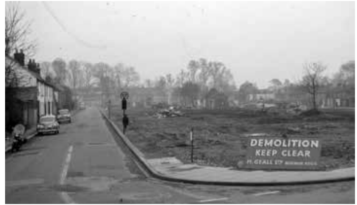
Demolition of properties in Somerstown
