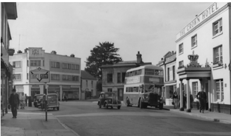
Central Buildings in the 1950s
