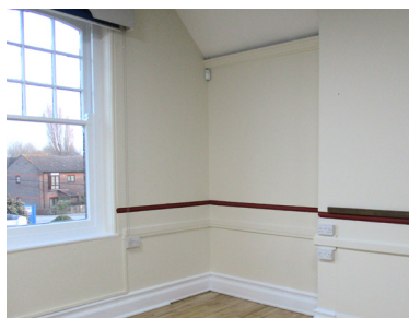
After the refurbishment
