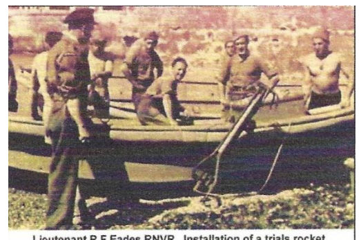
Lieutenant R F Eades RNVR. Installation of a trials rocket
